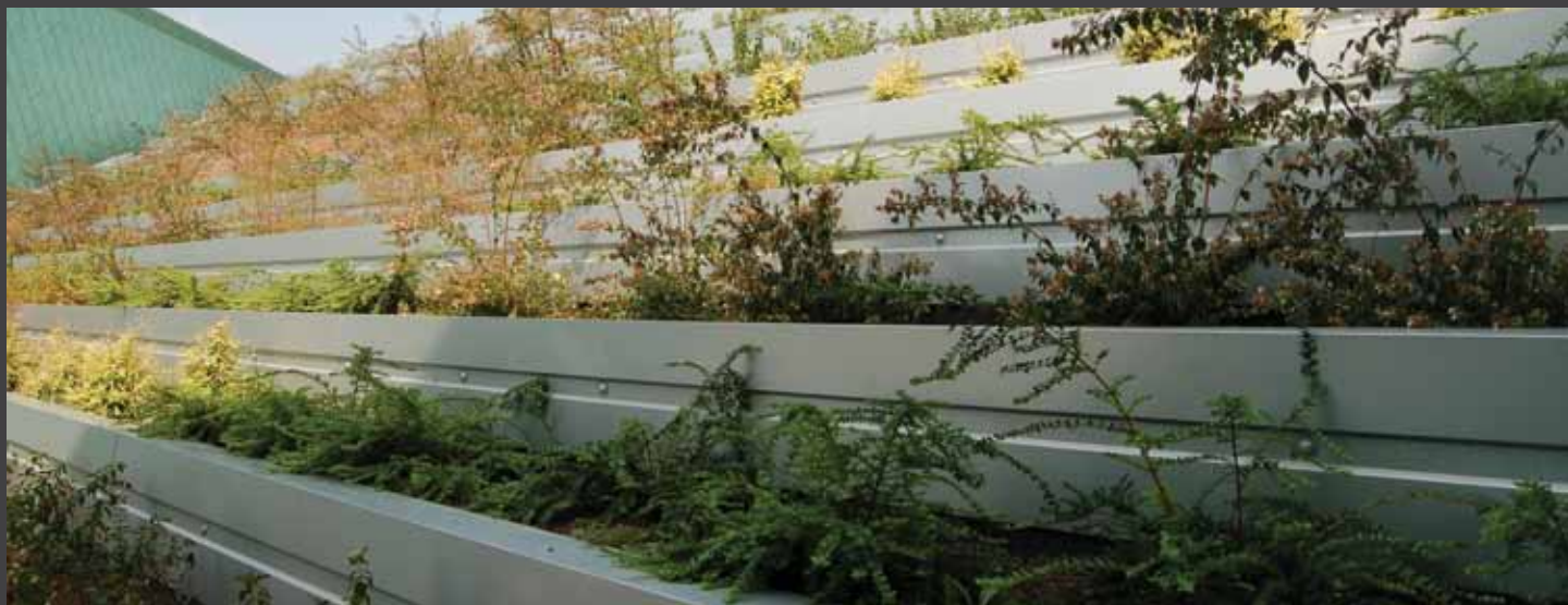
fig. 3) Giardino pensile "a terrazze" fruibile. Finished terraced green roof.
