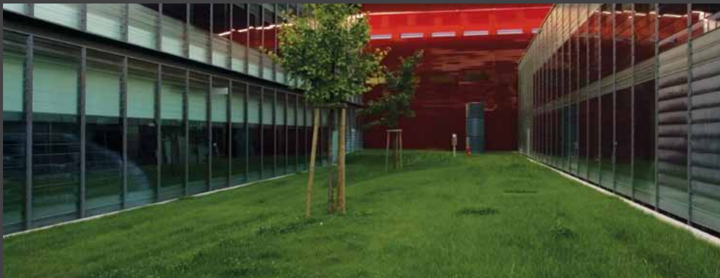
fig. 3) Aree verdi carrabili con GEOFLO® situate tra le strutture del Centro Ricerche Brembo S.p.A. Green surface suitable for vehicles made with GEOFLO®, Research Center of Brembo S.p.A.
